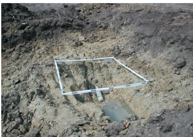
Ph.2 Location of detected 155 mm HE grenade in depth of 4 m from the excavation level
