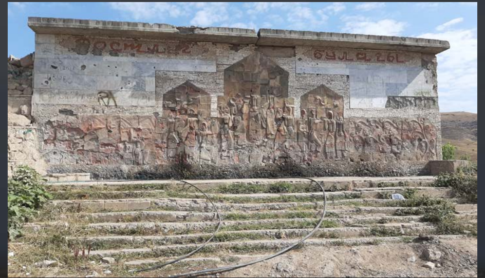
Abandoned "Dostluq" waterwell
